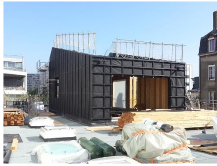
Extension ossature bois
